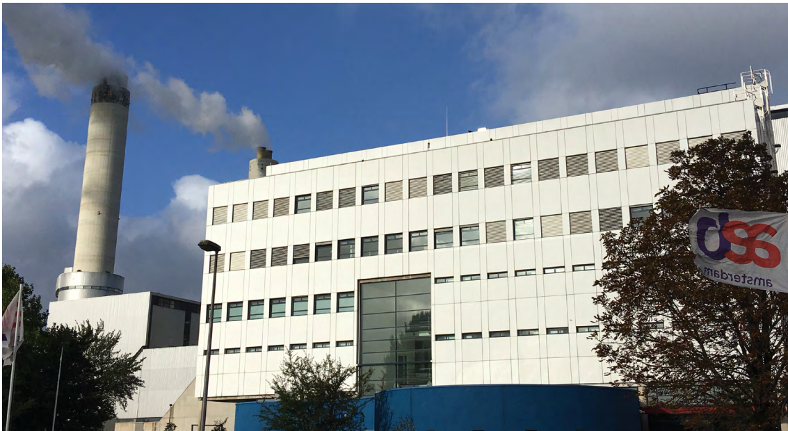
AEB Amsterdam Waste to Energy, The Netherlands
