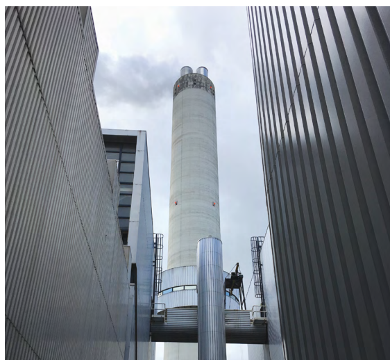
AEB Amsterdam Waste to Energy, The Netherlands
